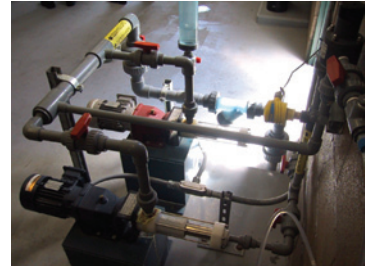
seepex pumps for NaOCl feeding into the discharge line of a vertical turbine pump
